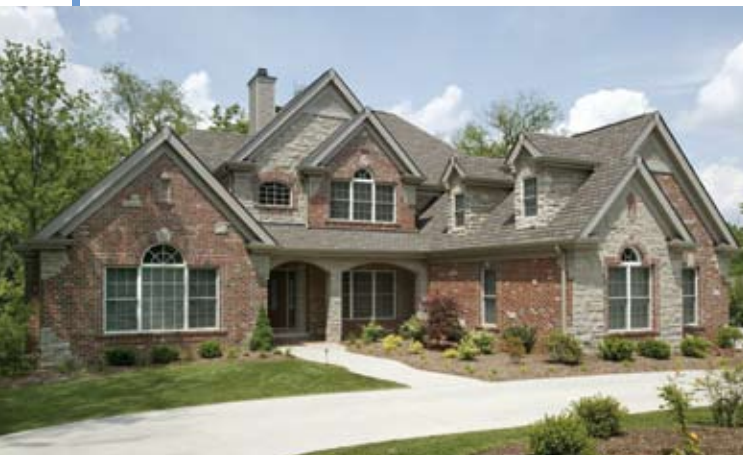
The homeowners decided to alter the plans slightly. They added the arches to the entry, dormers for additional light above the garage and different brick and stone exterior.
